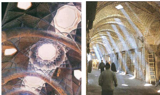
Fig.8: Ceiling openings in Kashan Baazar (left) Daylight in Raasteh (series of shops) Baazar (right)
