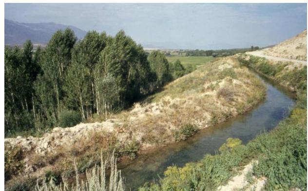
Figure 3 The 56 km long Samram canal, conveying water to the Urartian capital Tuspa (Vankale), from 800 BC.
