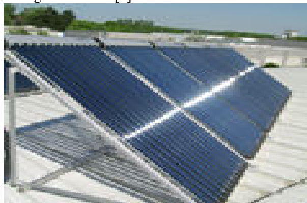
1: Installation of solar panels.
