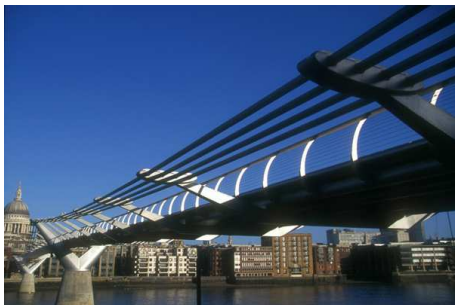
Fig. 1: Millennium Footbridge, London
