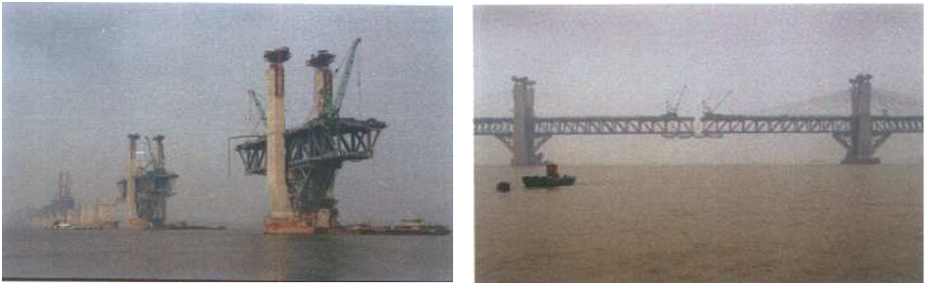
Fig.2 The construction photo of some cable-stayed bridge
