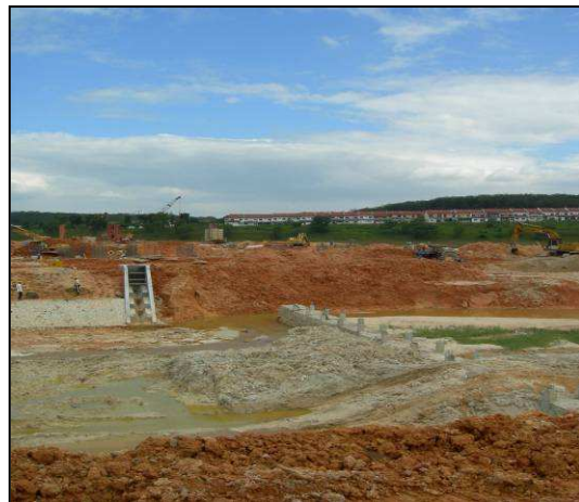
Fig.15: Drains from the new development Date: 30 January 2007
