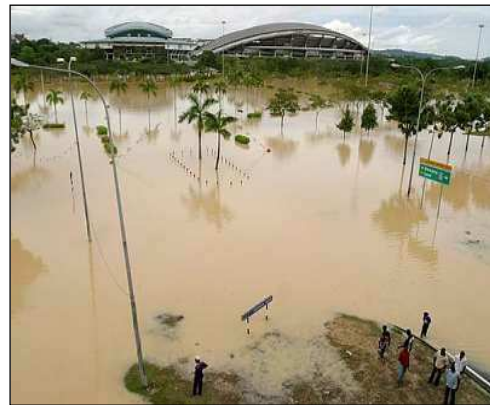
Fig.11: (Shah Alam Stadium)
