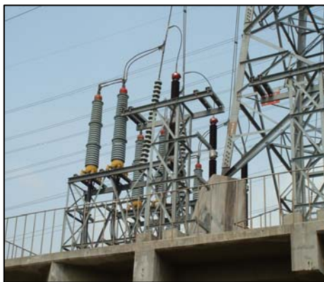
Fig.10 shows the foundation of cable connection station
