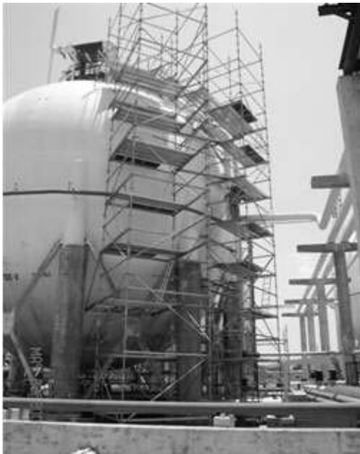
Fig. 1.- Spherical gas storage container with scaffolding for visual and ultrasonic inspection.
