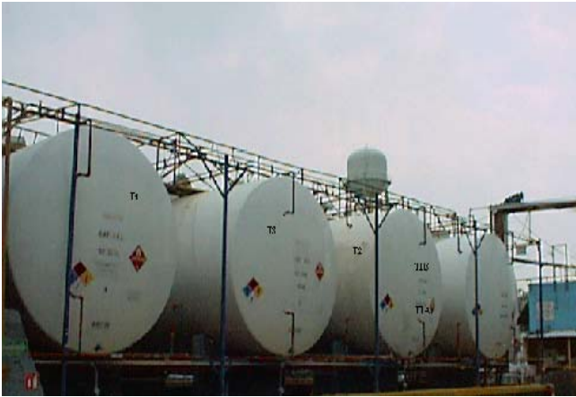
Figure 1 Horizontal cylindrical tanks from the Company Sherwin Williams. S. A. de C. V.
