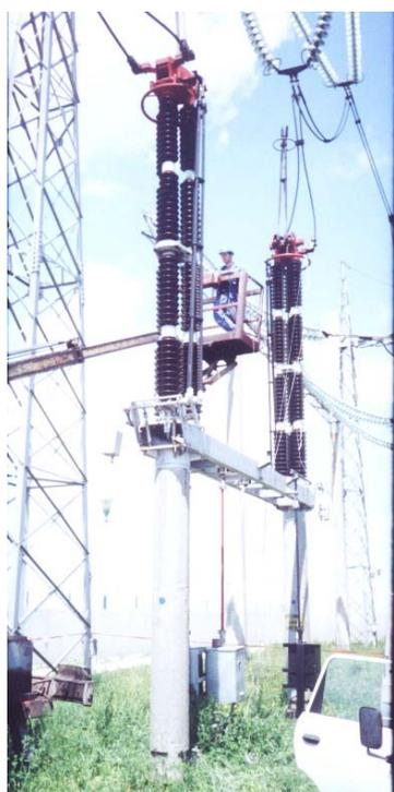
Fig. 1 The SMEP 400kV Disconnecter
