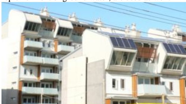
Figure 1: K2 sustainable apartments in Windsor, Victoria, Australia by Hansen Yuncken (2006) features passive solar design, recycled and sustainable materials, photovoltaic cells, wastewater treatment, rainwater collection and solar hot water. Source: Hansen Yuncken (2006)
