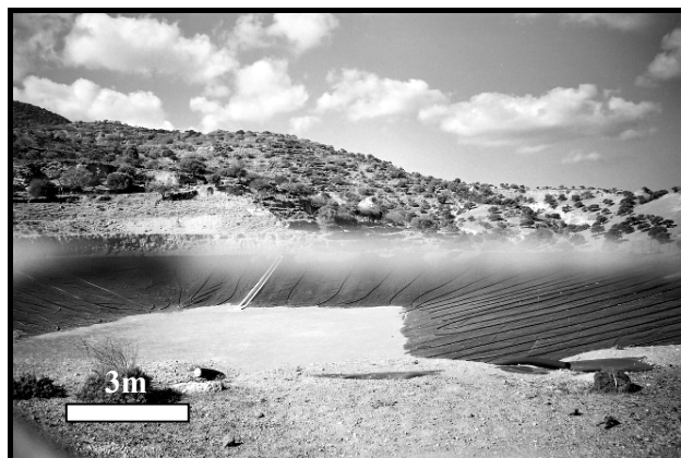
Fig. 4: Abandoned water reservoir of municipality of Nisyros in the vicinity of Hellinika near Katsouni Cape.
