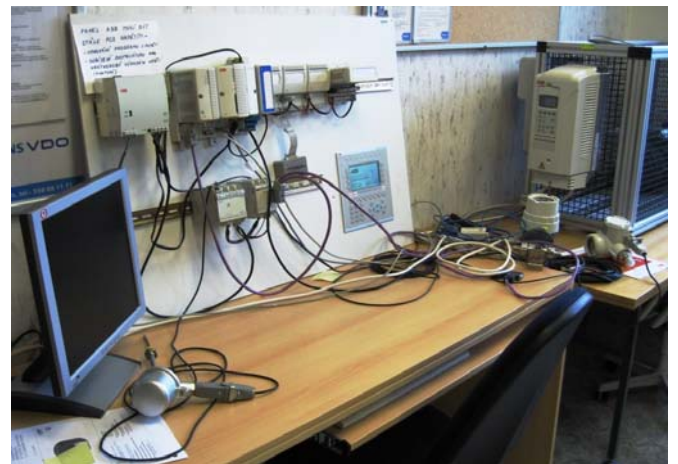
Fig. 7 Industrial modular PLC from ABB with Profibus DP Industrial LAN
