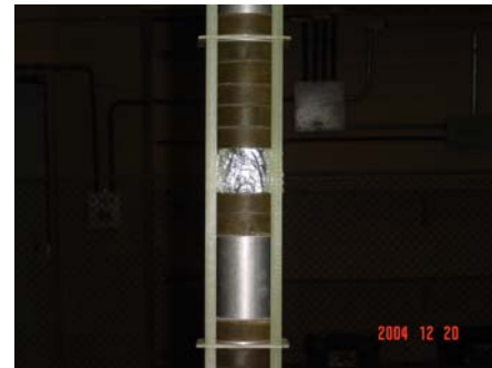
Fig. 5 – Short-circuited varistors in an arrester column.
