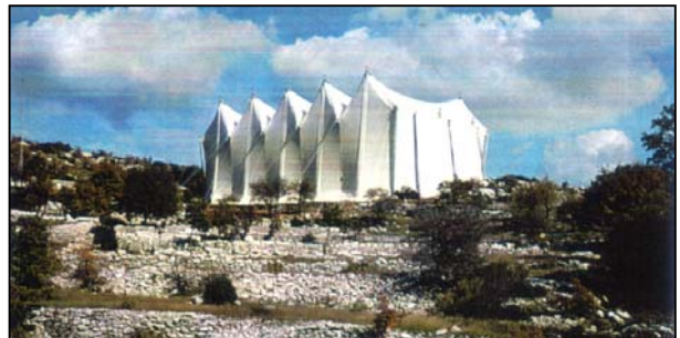
Fig. 10: Temporary coating around the Apollo's temple at Bassae
