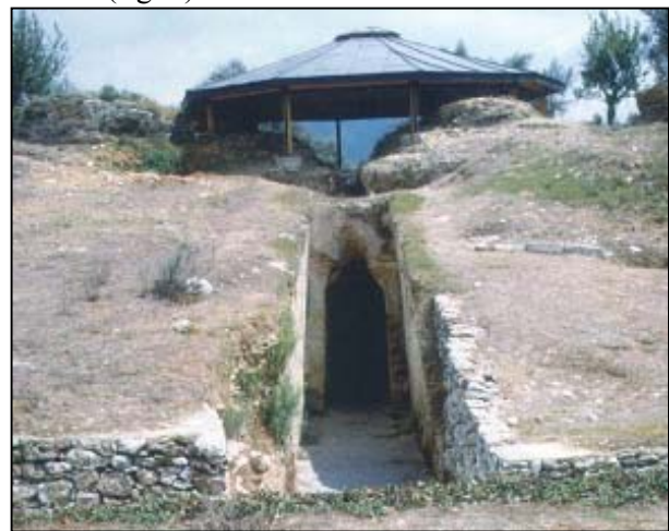
Fig. 2: The protection roof over the Mycenaean tomb in Pellana seen from the entrance corridor
