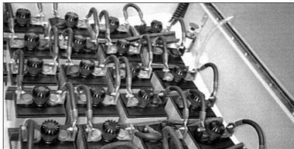
Fig.7 – Connections of batteries arrays
